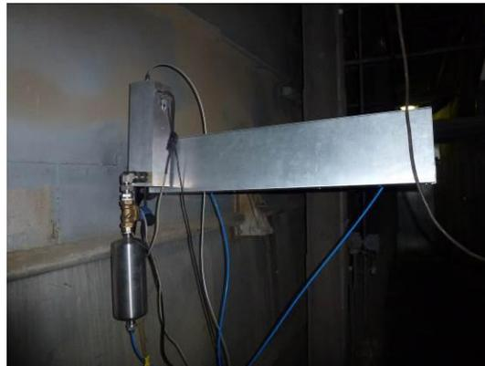
**Figure 2.** The analyser mounted on the wall of the boiler
